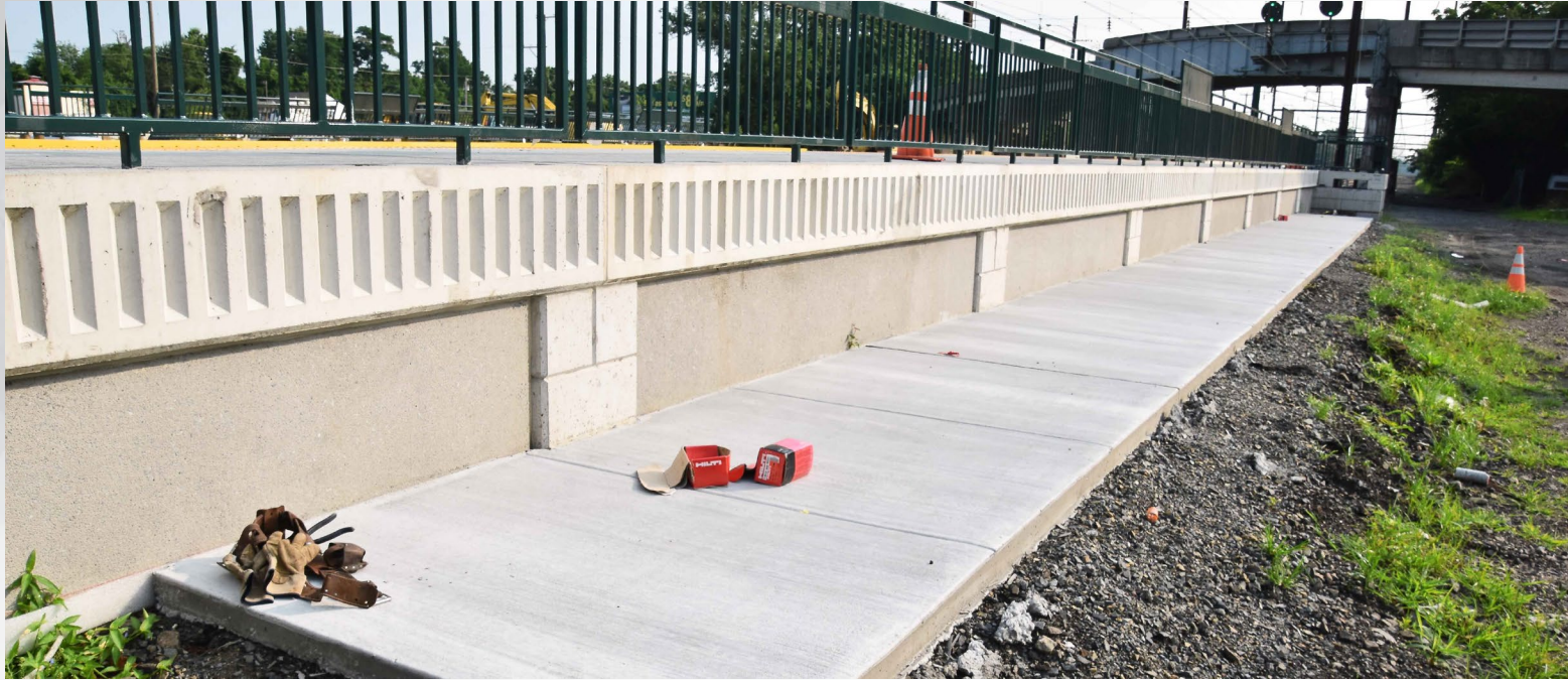
Precast infill panel closes off gap and prevents trespassing
