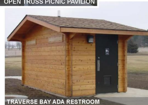
TRAVERSE BAY ADA RESTROOM
